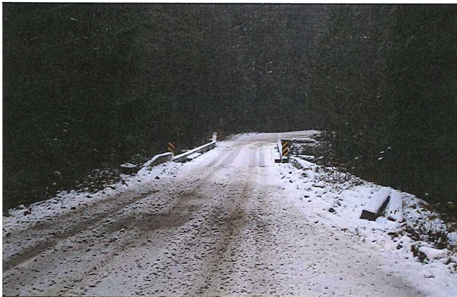
CK-2031 Approach Right Bank
