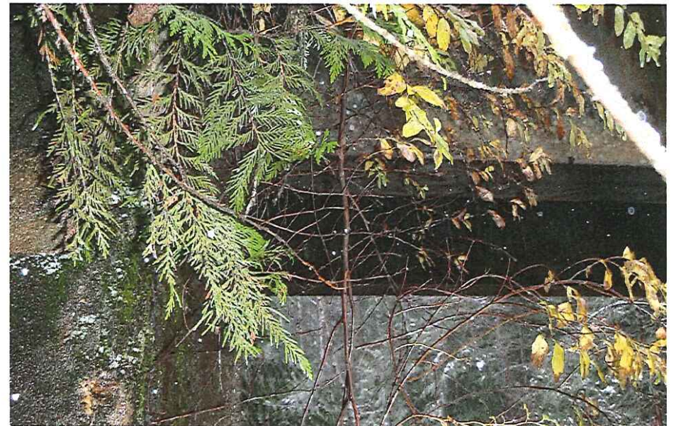
CK-2031 Abutment Left Bank
