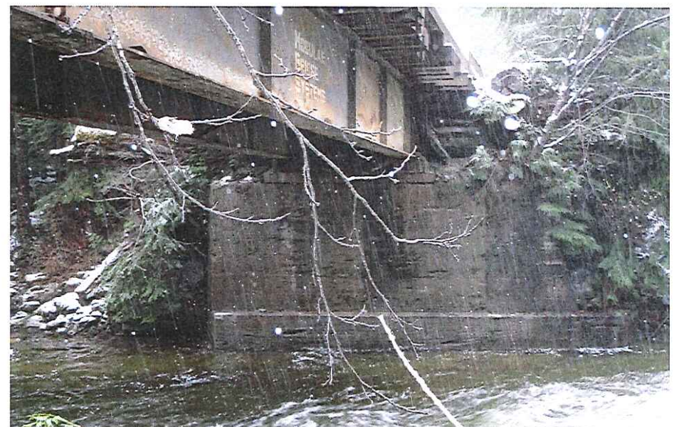
CK-2031 Abutment Right Bank
